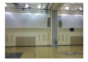
Here we see a motorized overhead storage system for arrow nets. It is operated with a key switch. Manufacturer is unknown.
