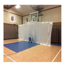
In some gyms maintenance staff have installed heavy duty eye bolts (or metal plates) in the walls to create the needed attachment points They are installed at about 9 feet high and 30-36" away from any adjoining wall so that the minimum 30" clearance behind the arrow curtain is maintained. Sagging of the net (in some cases) is eliminated via a support hung from the backboard.
